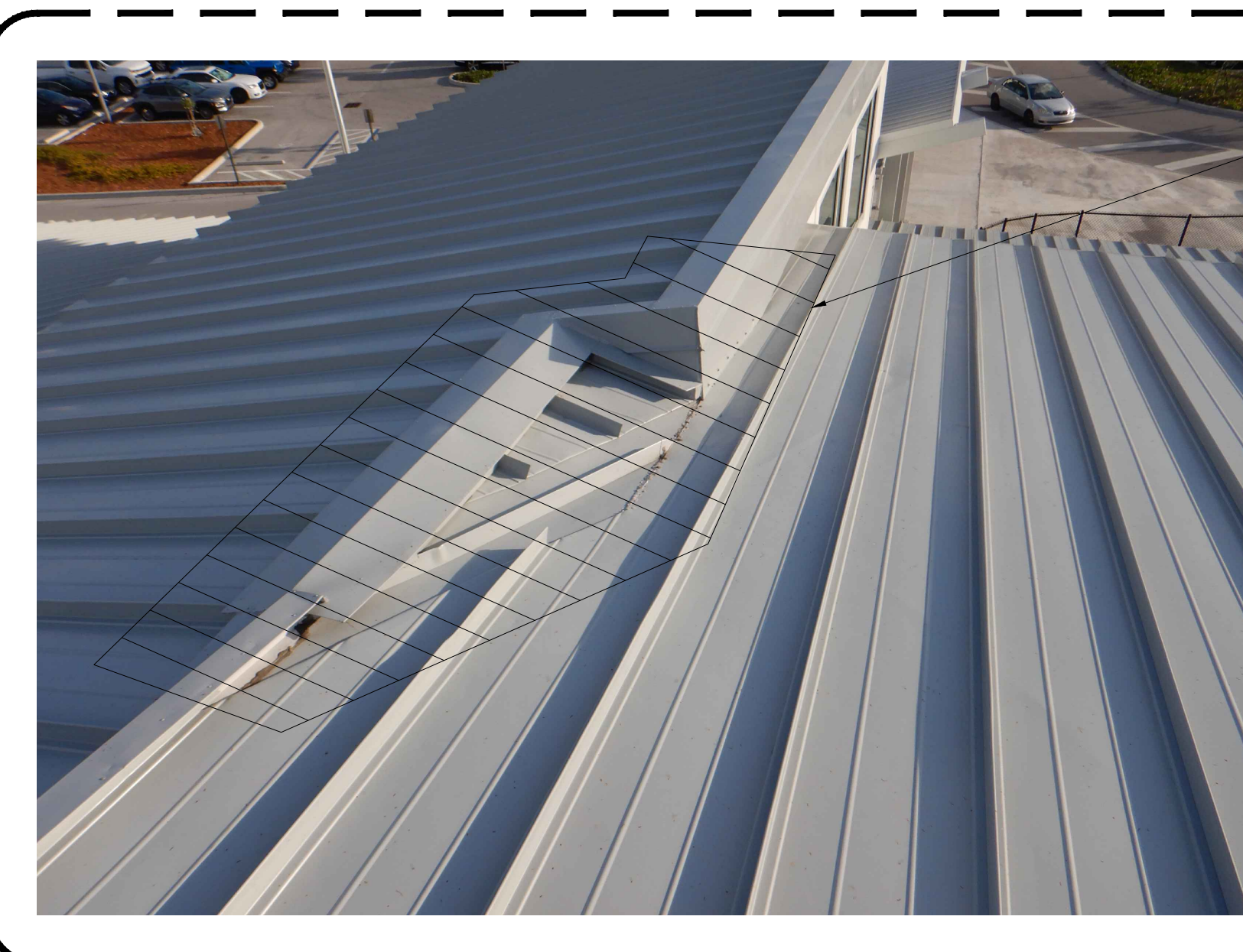
D REPAIR AREA #6 PHOTOGRAPH SCALE: NTS
