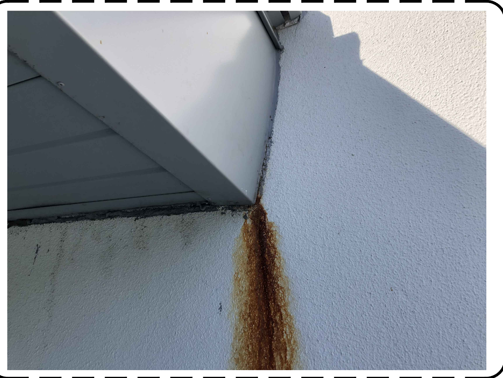
I REPAIR AREA #7 PHOTOGRAPH SCALE: NTS
