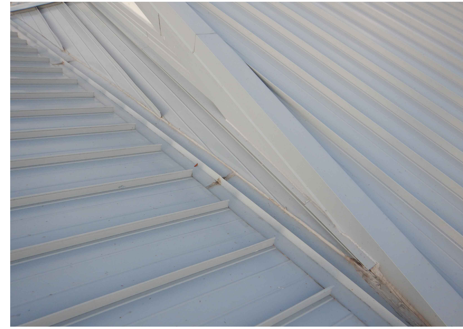
C PHOTOGRAPH OF REPAIR AREA #1 SCALE: NTS
