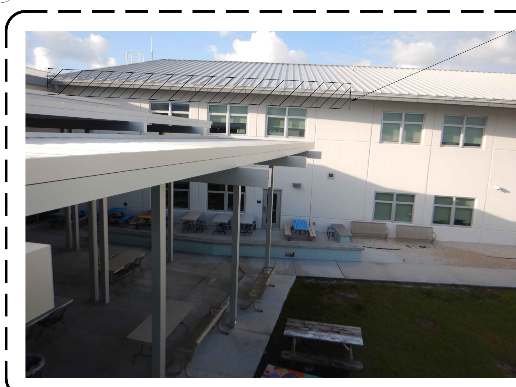
E BUILDING ENVELOPE REPAIR ITEM #2 PHOTOGRAPH A5.1 SCALE: NTS
