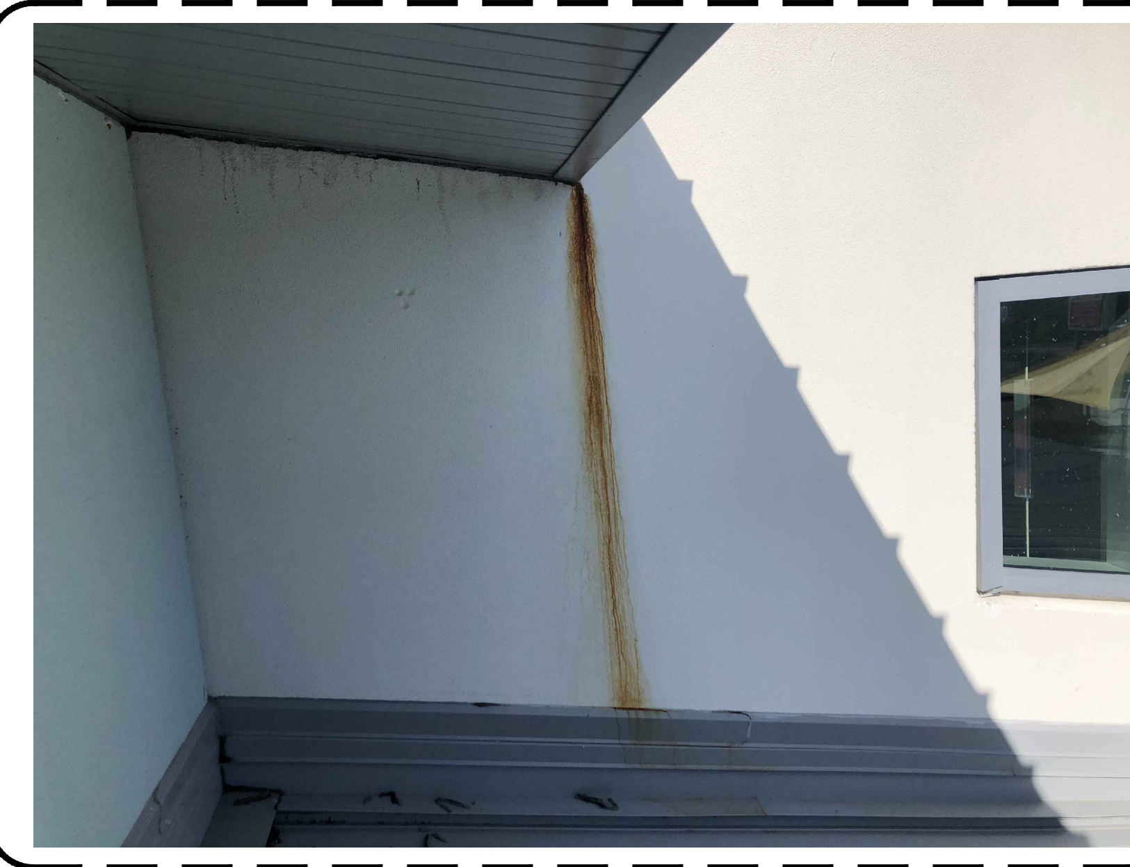
G REPAIR AREA #7 PHOTOGRAPH SCALE: NTS
